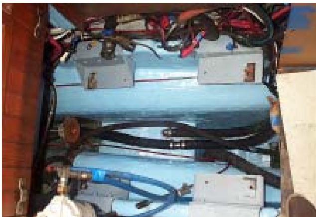
Looking down: port side of engine foundation is at top of photo.
