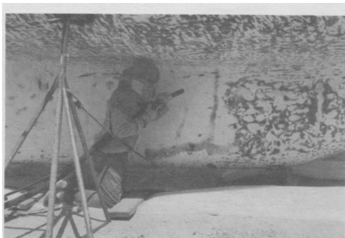
SANDBLASTING GETS TO CLEAN GEL-COAT. First pass removed all paint and barnacles, as shown above right. Second pass being made opens all blisters to begin the drying process.
